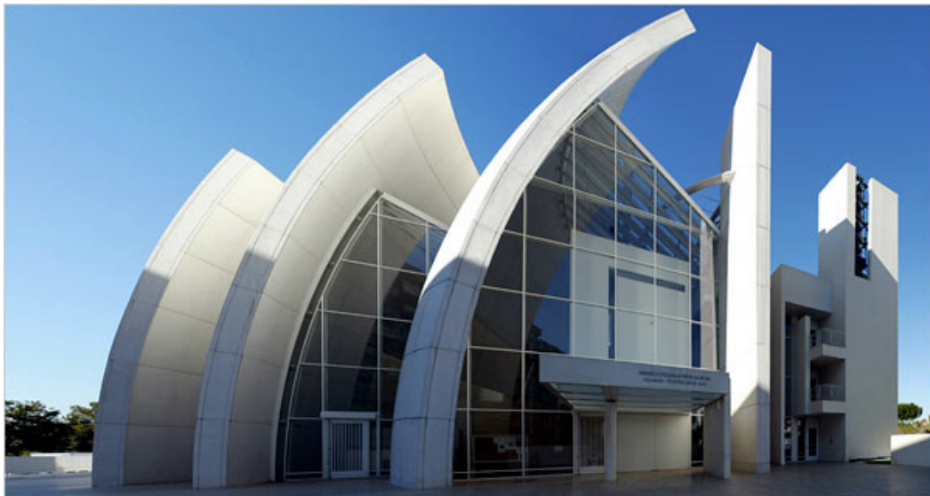
The soaring structure of the Jubilee Church in Rome, designed by American architect Richard Meier, is made from precast concrete elements coated with Italcementi's TX Active cement. There is a stark contrast between the brilliant white surfaces of the overall structure and the dirty, gray joints which were not treated with the \text{TiO}_2 product. Photo credit Yusheng, Liao. November 2006.
